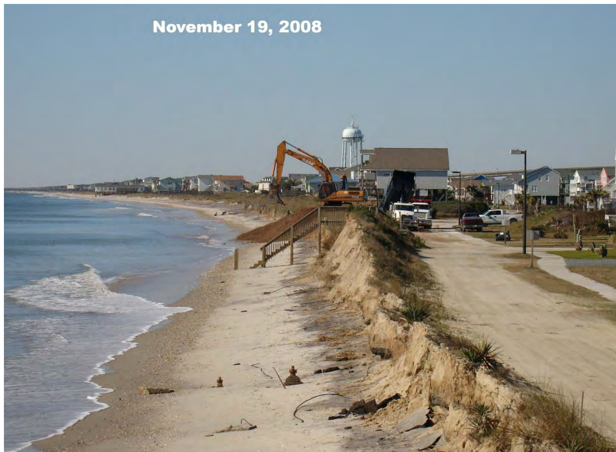
Figure 1-4. Holden Beach East End Dune Restoration Activities Following Hurricane Hanna Dune Erosion and Breaching
