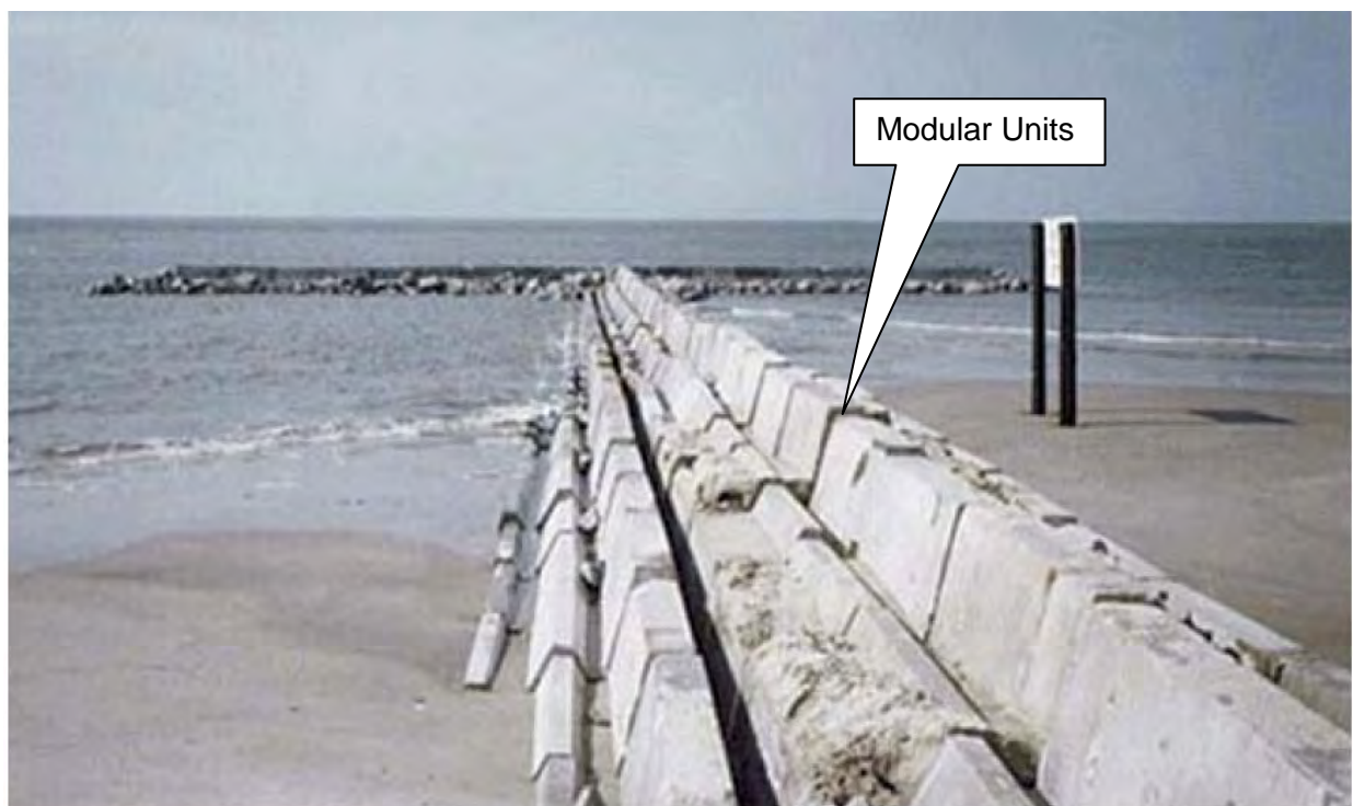
Figure 8-10. Tybee Island, Georgia Terminal Groin Structure that was Successfully Modified by Removing Six Modular Units on the Seaward End (source: USACE, 1997). Also note T-Head feature.
