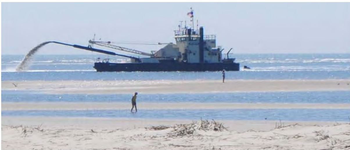
Figure 4-5b. Merritt Sidecasting Dredge Working the LWF Outer Channel in Spring 2012. “Deep water” channel orientation is closer to the Holden Beach shoreline for this particular event.
