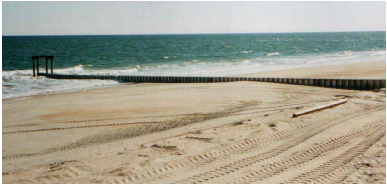
Figure 8-1. Garden City, South Carolina, Sheetpile Groin after Construction during Low Tide (photo date: January 2003)
