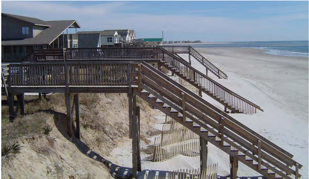
Figure 9-4. March 2010 Photo at Station 30+00 Looking East. Scarped dune conditions are typical for this reach.
