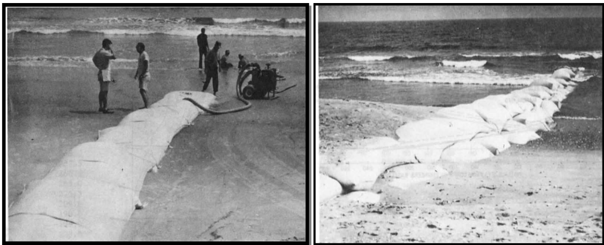
Figure 4-17. Groin Construction and Placement in 1970s (source: Machemehl, 1975b)
