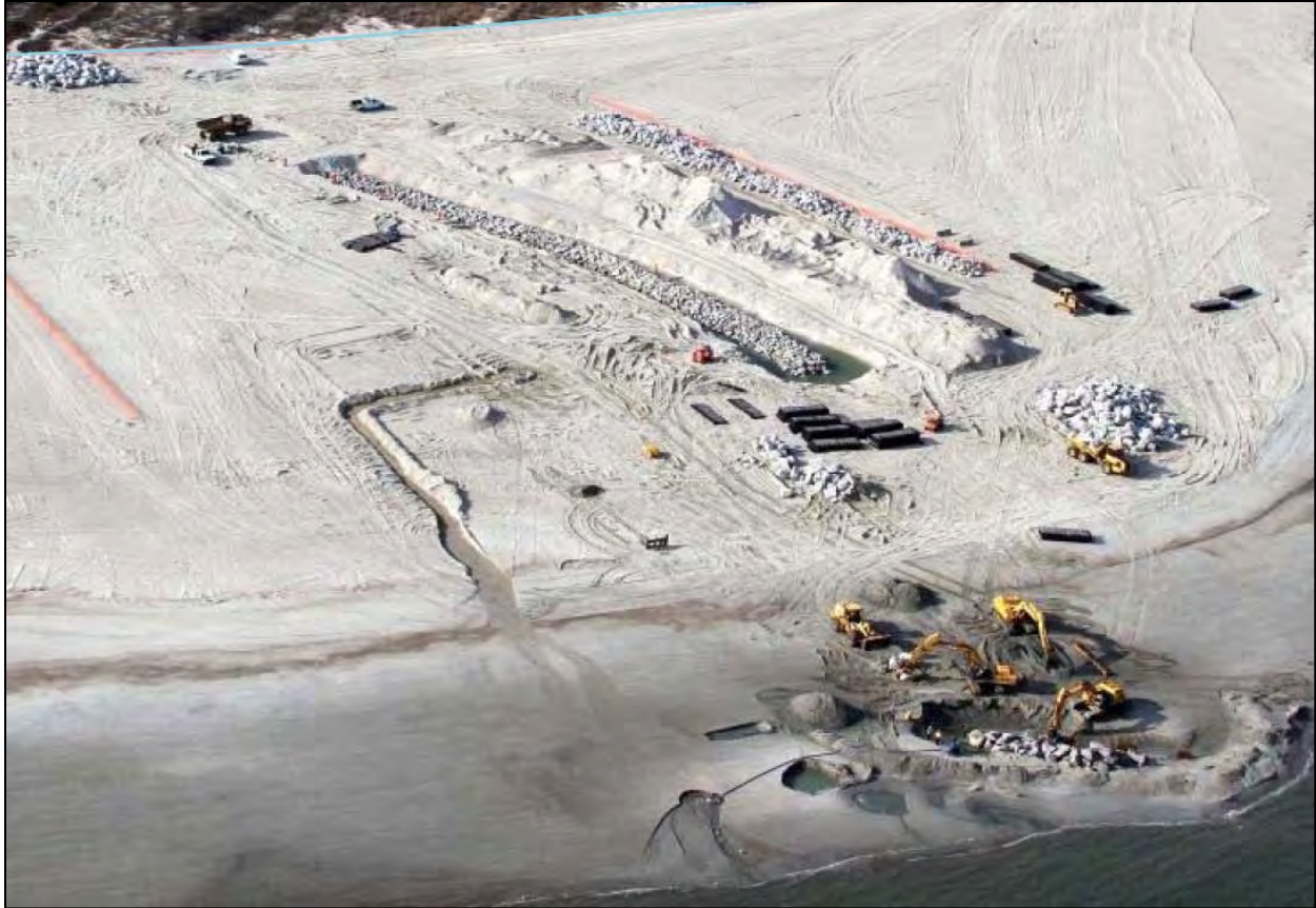
Figure 8-4. Recently Installed “Leaky” Terminal Groin on Hilton Head, SC during construction. Groin was constructed with only armor stone (no core stone was used) in 2012 (source: Olsen Associates).
