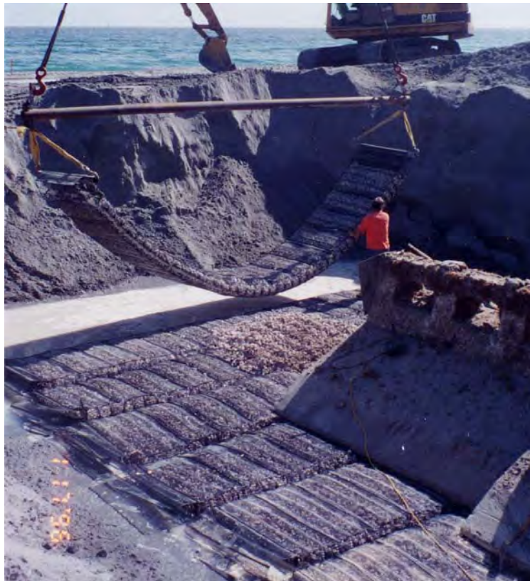
Figure 8-3a. Groin Construction Showing Mattress Placement
