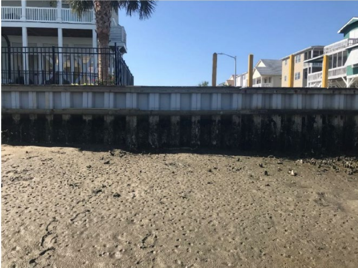
Figure 6. Existing Vinyl Sheetpile Wall (Cobia Street)
