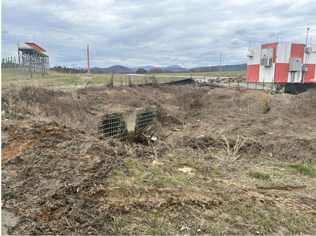
Photo 1. Upstream end of existing culvert
