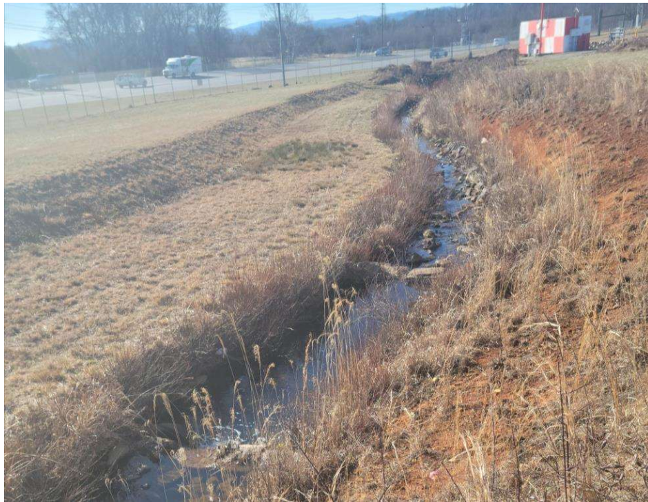
Photo 4. Land uses upstream of existing culvert (facing downstream).
