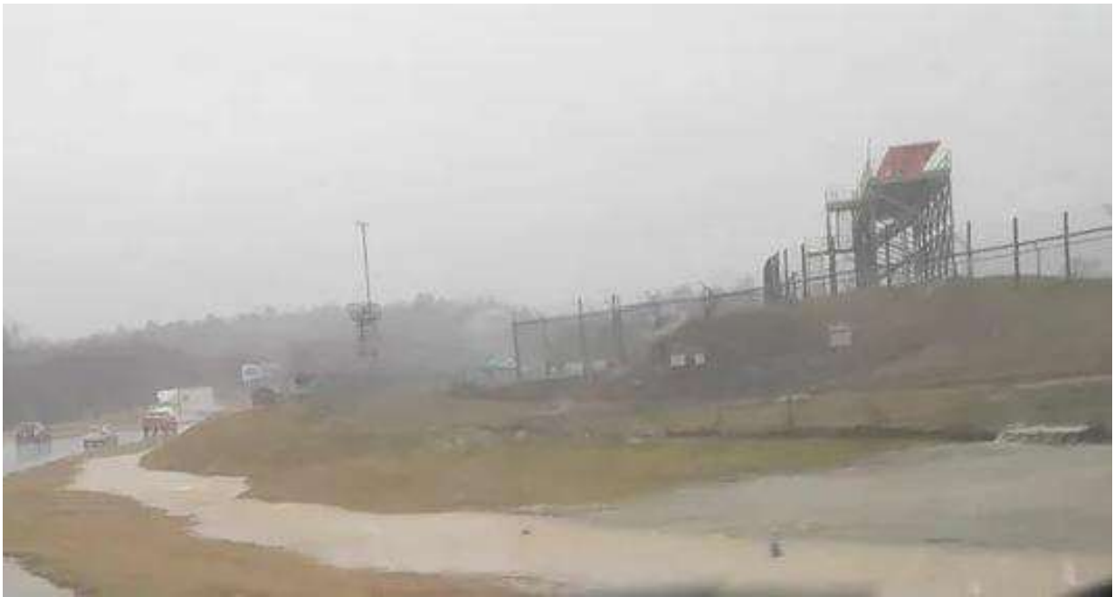
Photo 2. Flooding resulting from clogged culvert grate
