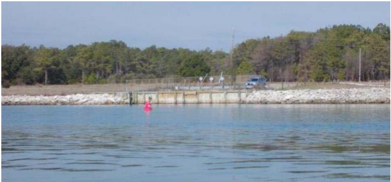
Photo C-2: Shoreline armoring to prevent erosion along mainland LWF Inlet shoreline (vehicle in photo is parked at the end of Stone Chimney Road).
