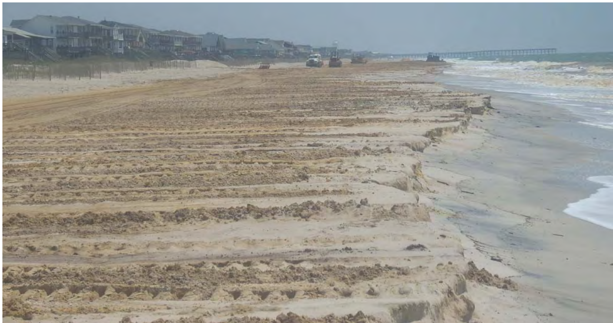
Figure 7-4: 2009 Holden Beach Nourishment Project during Construction (West Reach is shown). Typical upland placement that will be employed for the proposed terminal groin project.
