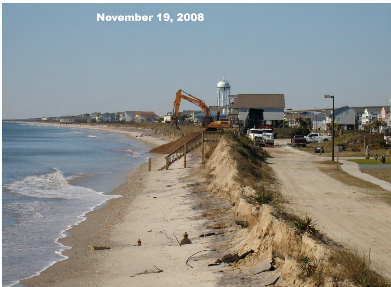
Figure 2-1: Holden Beach East End dune restoration activities following Hurricane Hanna dune erosion and breaching.
