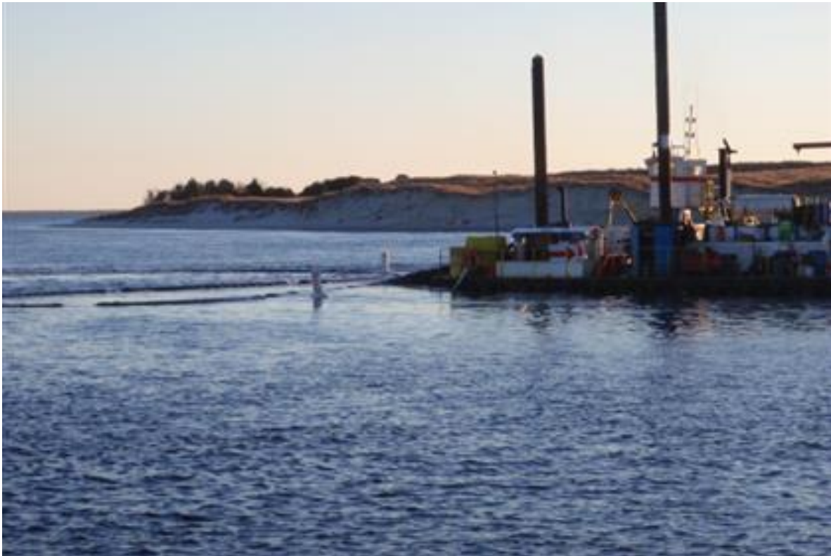
Photo 3.1. Pipeline dredging of the AIWW Bogue Inlet crossing.
