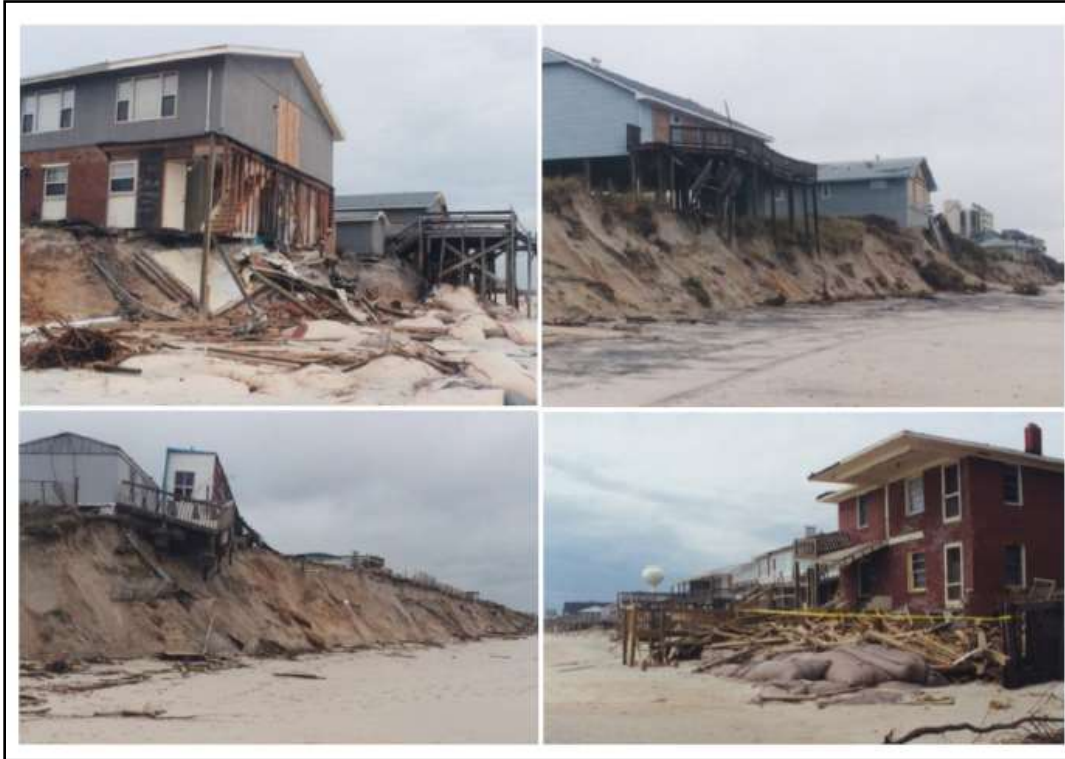
Photo 2.1. 1990s hurricane damage.
