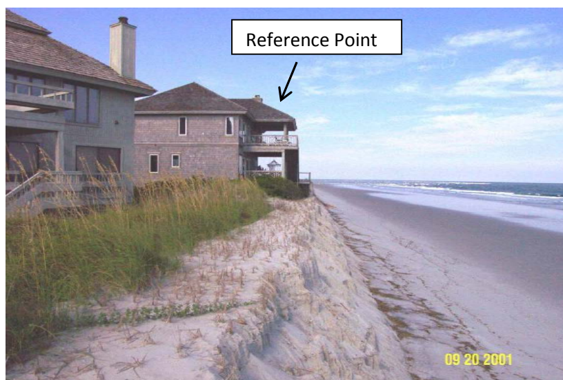
Figure 2.7. Evidence of rapid erosion approximately one month following 2001 nourishment
