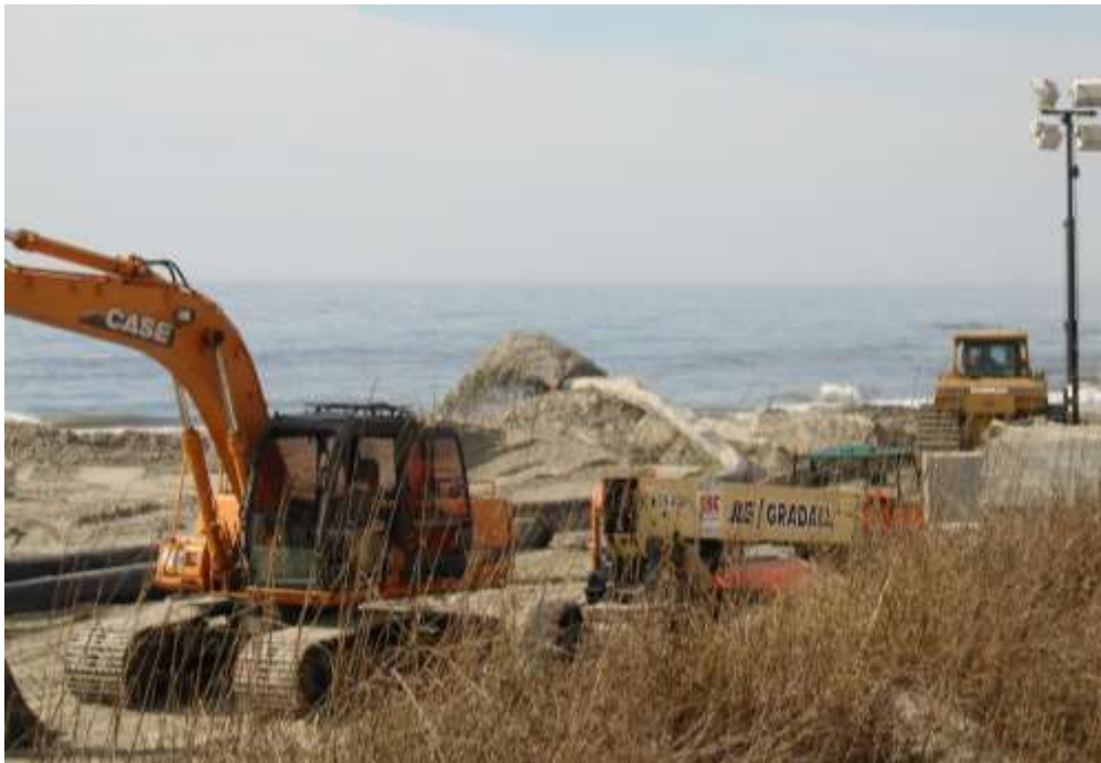
Photo 3.2. Equipment utilized during the 2014 beneficial use project on the East End.
