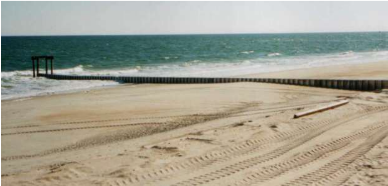
Photo 3.4. Garden City, SC, sheet-pile groin after construction during low tide
