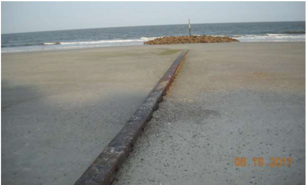
Photo 3.5. Hunting Island SC groin at low tide.
