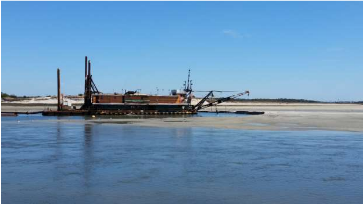
Photo 5.1. The dredge Marion working in Eastern Channel, spring 2015.
