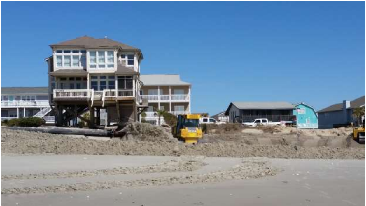
Photo 5.2. Sand placement activities on the west end of Oak Island, spring 2015.
