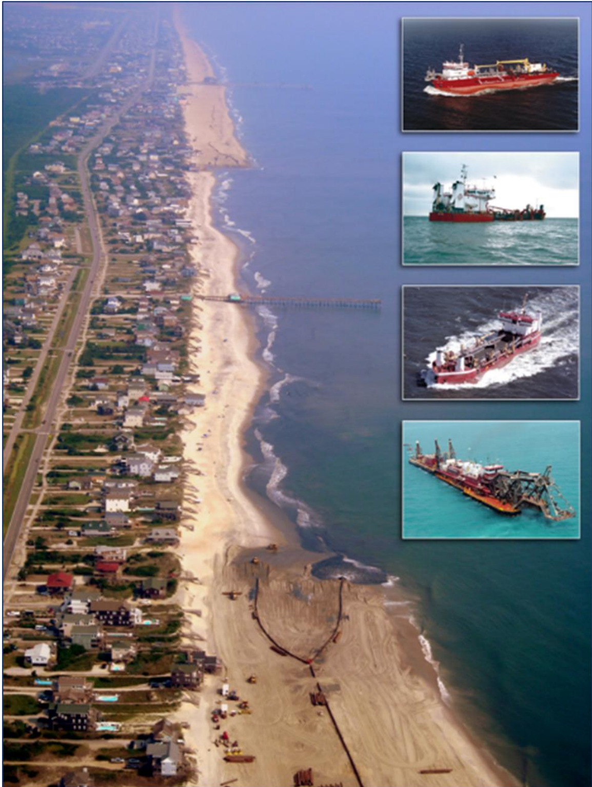
FIGURE 3.11. Three hopper dredges and one suction cutterhead dredge (inset photos) were used to construct the Nags Head (NC) beach nourishment project (24 May to 27 October 2011). Image shows nourishment construction in progress working south to north toward Outer Banks Pier in south Nags Head. [Photos by CSE and Great Lakes Dredge & Dock Co.]
