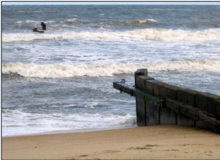
FIGURE 8.5. Cape Hatteras Groins. [UPPER] Groins 2 and 3 on 4 November 2013. [MIDDLE LEFT] Groin 3 – wing wall with Hatteras Lighthouse in the distance on 19 March 2013. [MIDDLE RIGHT] Groin 1 – visible remnant section in the surf zone on 19 March 2013. [LOWER] Groin 2 – missing sheet piles, damage and deflection at seaward end on 4 November 2013. [CSE 2013]
