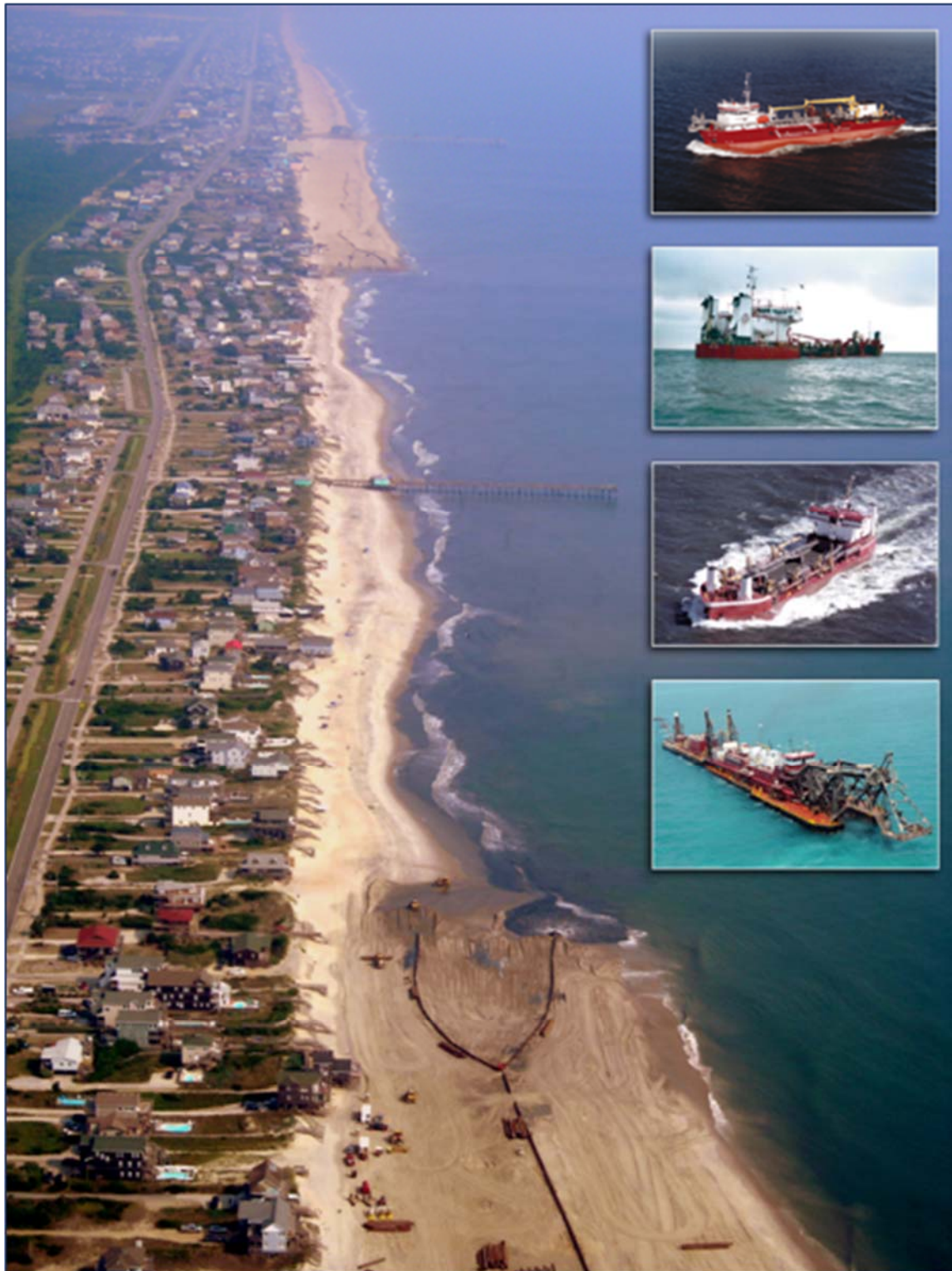
FIGURE 3.6. Three hopper dredges and one suction cutterhead dredge were used to construct the Nags Head (NC) beach nourishment project (24 May to 27 October 2011). Nourishment construction in progress working south to north toward Outer Banks Pier in south Nags Head. [Photos by CSE and Great Lakes Dredge & Dock Co]
